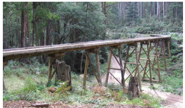
15000' Siphon trestle bridge, named because of its distance in feet from the beginning of the tramline at the top of the haulage, has been reconstructed to original specifications
